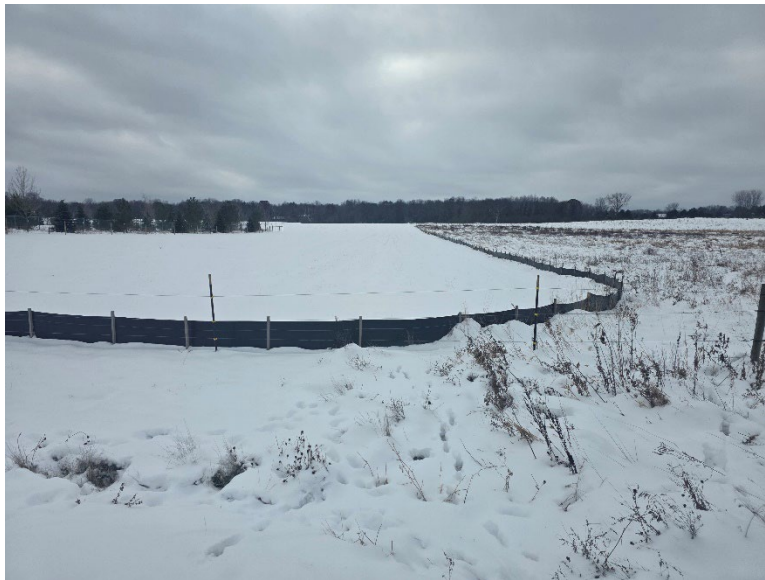
Facing south near MP 0.10, silt fence is functional, and site is snow covered.
