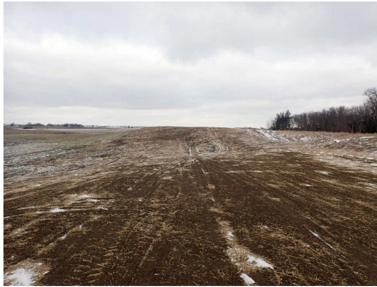
Facing north at MP 31.45, south of 140th Street and north of 135th Street, temporary workspace is seeded with Minnesota CP1, mulched and crimped.
