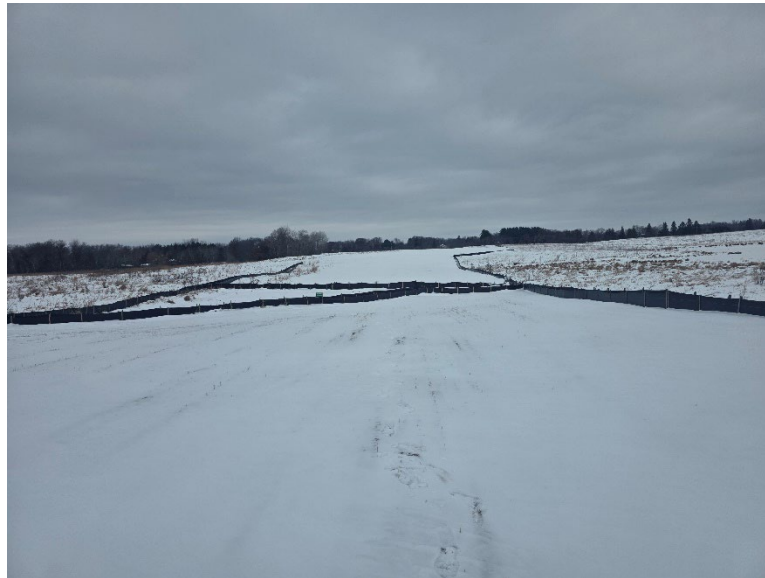
Facing north near MP 1.35, silt fence protecting wetland FRM-W13 is functional, and site is snow covered.
