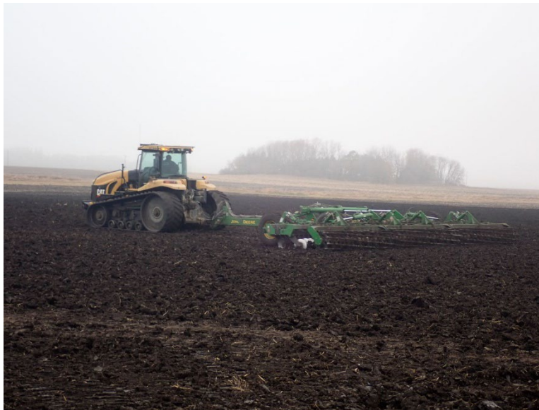
Facing north at MP 34.20, K&K decompacting topsoil at the staging area north of 165th Street.
