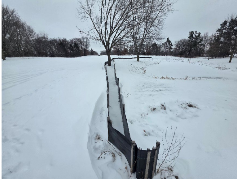
Facing east near MP 2.40, redundant silt fence is in good condition and site is snow covered.
