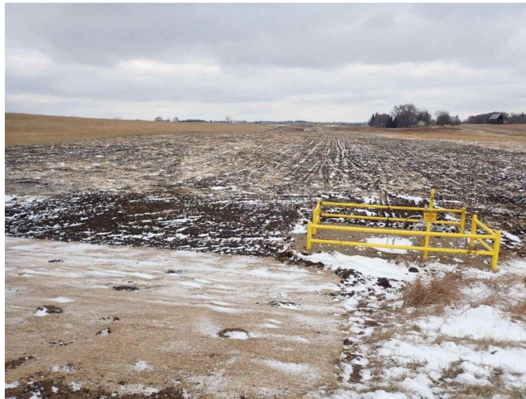
Facing north at MP 31.20, north of 135th Street, temporary workspace seeded with Minnesota CP1, mulched and crimped. Roadside ditch (temporary access road) seeded with Minnesota DOT 24-151 (General Roadside) and ECBs installed.
