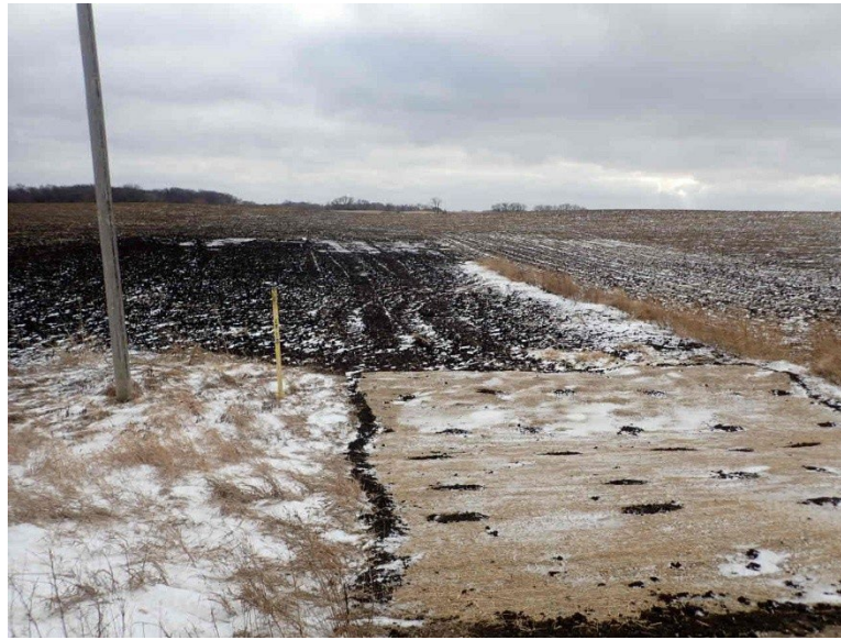
Facing south at MP 31.2, south of 135th Street, decompacted temporary workspace. Roadside ditch (temporary access road) seeded with Minnesota DOT 25-141 (General roadside) and ECBs installed on roadside ditch (temporary access road).
