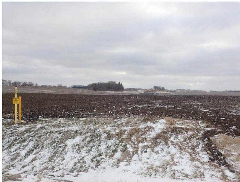
Facing south at MP 31.95, south of 140th Street, decompacted temporary workspace. Roadside ditch (temporary access road) seeded with Minnesota DOT 25-141 (General Roadside) and ECBs installed on roadside ditch (temporary access road).
