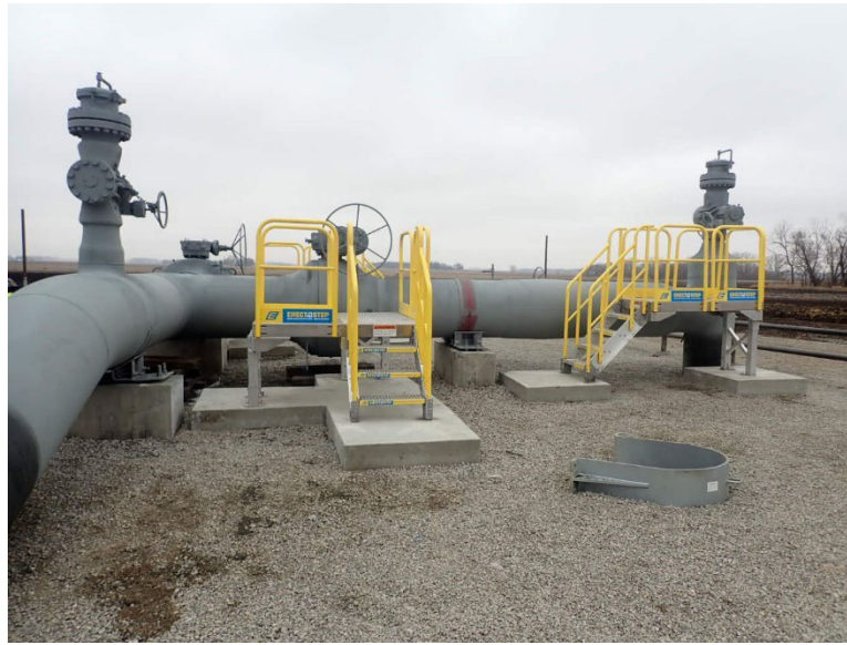
Facing north at MP 34.20, K&K completed abrasive blasting and painting operations for the aboveground valve setting north of 165th Street.
