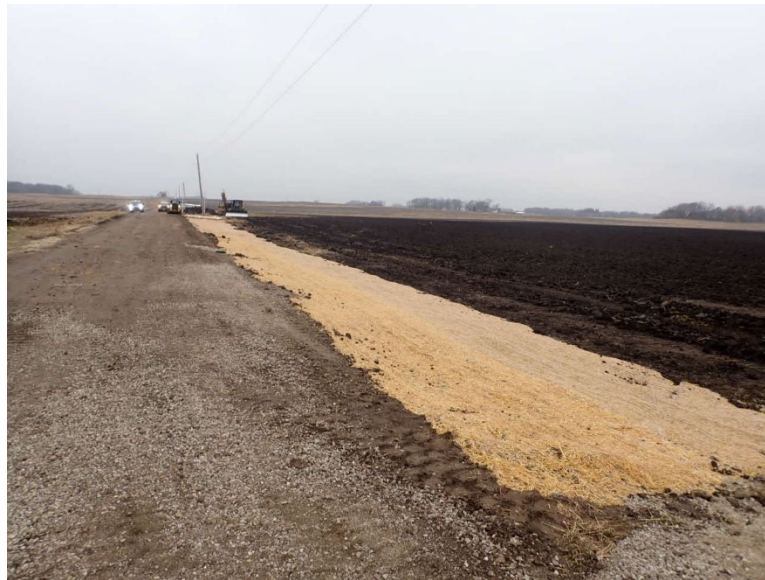
Facing northwest at MP 34.20, K&K completed installation of permanent erosion control devices (ECDs) for the roadside ditch (temporary access road for the staging area) north of 165th Street.
