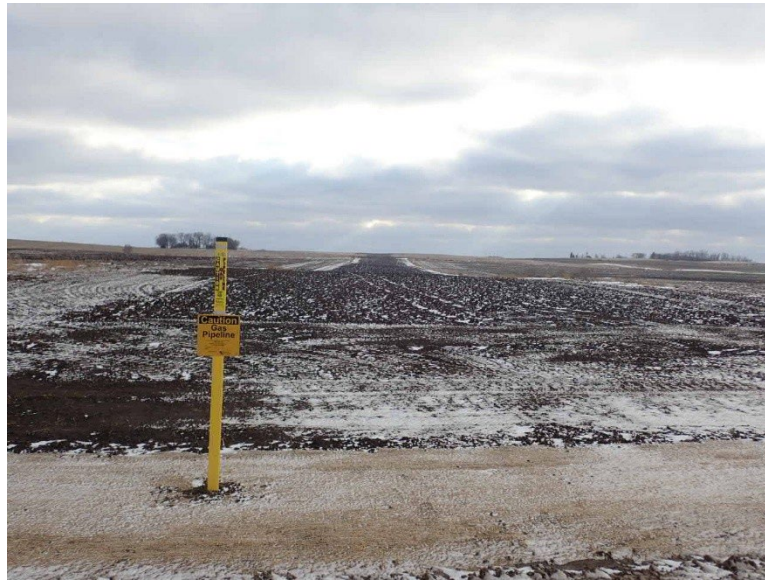
Facing south at MP 34.20, decompacted temporary workspace south of 165th Street. Erosion control blankets (ECBs) installed on roadside ditch (temporary access road).
